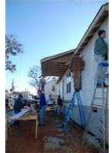
Keeping those posts level for solid start to the decking
